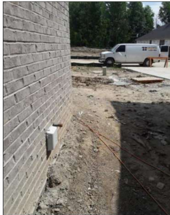
Clear pathway from meter location to street.
