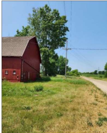
Approved overhead permanent service and clear path.
