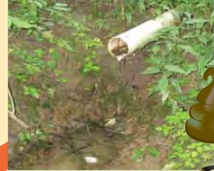
Sewage pollutes rivers and lakes when people have septic tank overflow pipes or improperly dump travel trailer or porta-potty waste. You can tell when sewage is present - it has a distinct odor. There may also be black staining inside the drainage pipe and visible evidence of sanitary waste, such as toilet paper and opaque or gray water.
