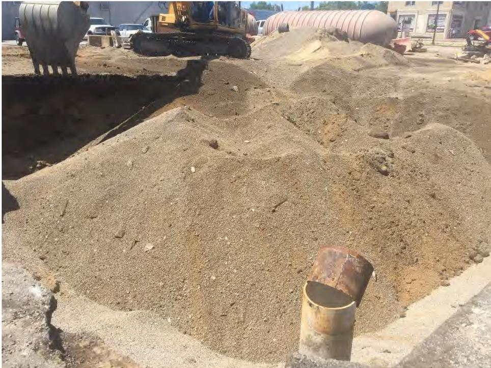
Photograph 12: View of gasoline UST cavity backfill in progress.
