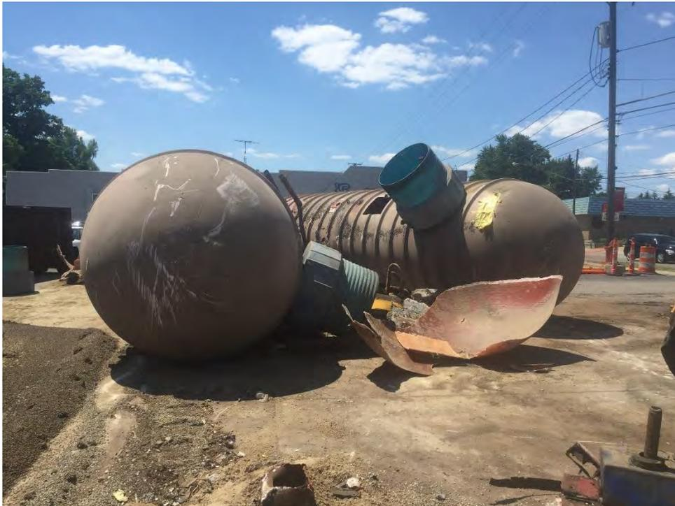
Photograph 10: View of removed gasoline USTs being dismantled.
