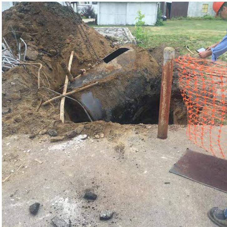
Photograph 6: View of removal of heating oil UST.
