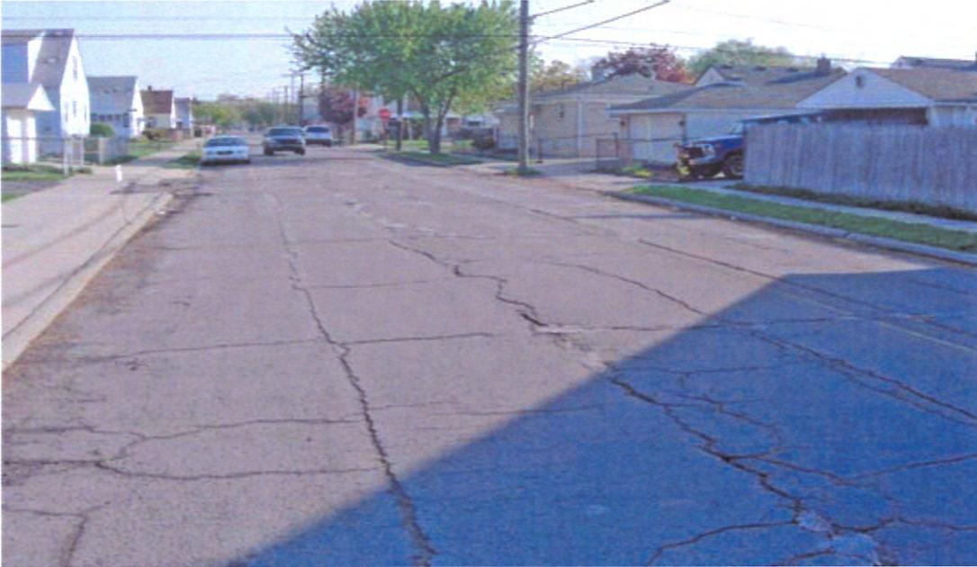
**Lafayette St in Lincoln Park was first milled to improve the ride. This is not always necessary. A single chipseal was applied using CM-90 asphalt and 29a slag aggregate in May of 2008.**
