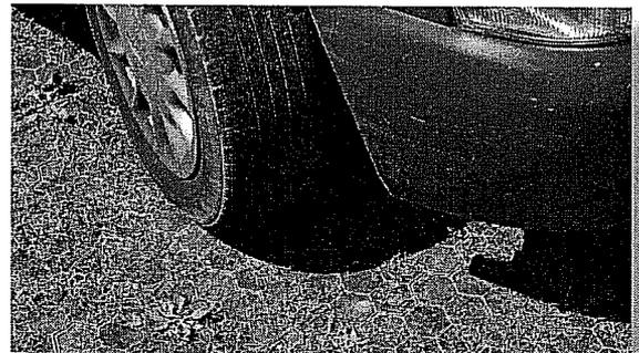
*This driveway with permeable/porous covering helps reduce polluted runoff by allowing stormwater to soak into the ground.*
